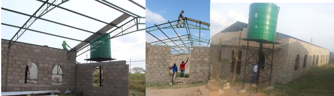
Church with the roof being installed and walls closed up!
